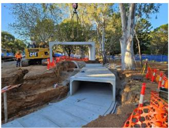
The project involves the replacement of the existing twin cell culvert beneath Unley Road that facilitates the flow of Park Lands Creek from Park 19 into Park 20. The existing culvert is in poor condition with walls being held up by props at the western end.
